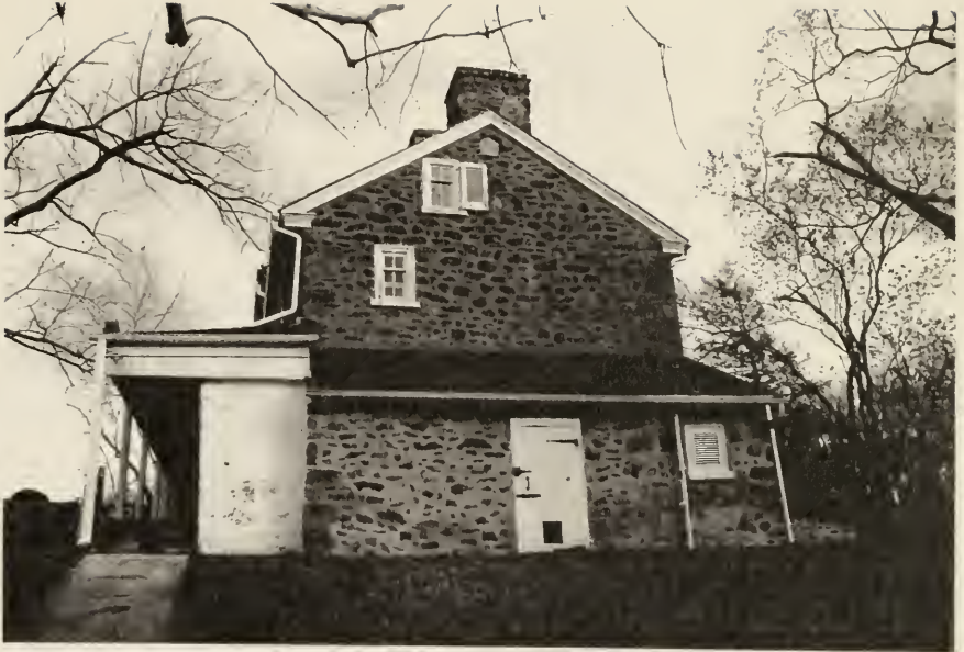
Figure 15. West elevation of kitchen wing showing "June 1765" datestone and the later smokehouse addition. (1994)
